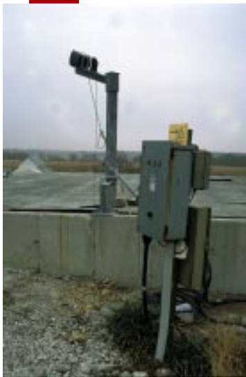
The digester tank at Bell Farms.
